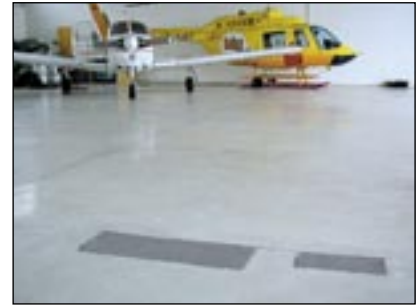
Mannheim Airport Repairing hangar floors
