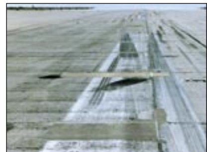
Leipzig/Halle Airport: Repairing concrete, runways and taxiways
