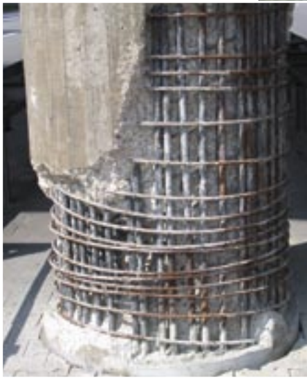
Repairing a concrete pillar damaged by de-icing salt
